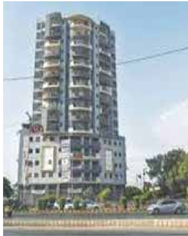
Nasla Towers Being Demolished
