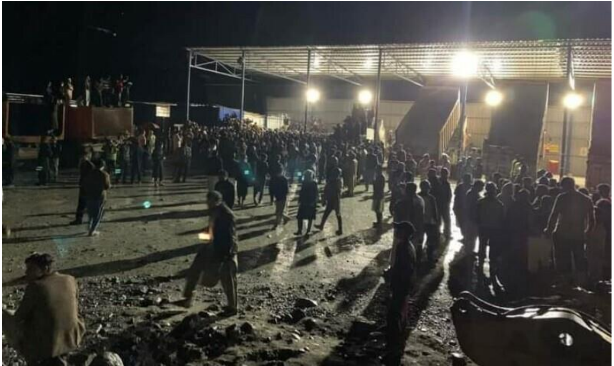
The photo shows the Dasu dam site.
